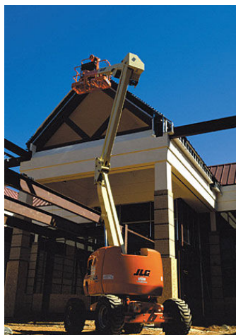
Kerr's JLG 450AJ 45ft Boom Lift.
